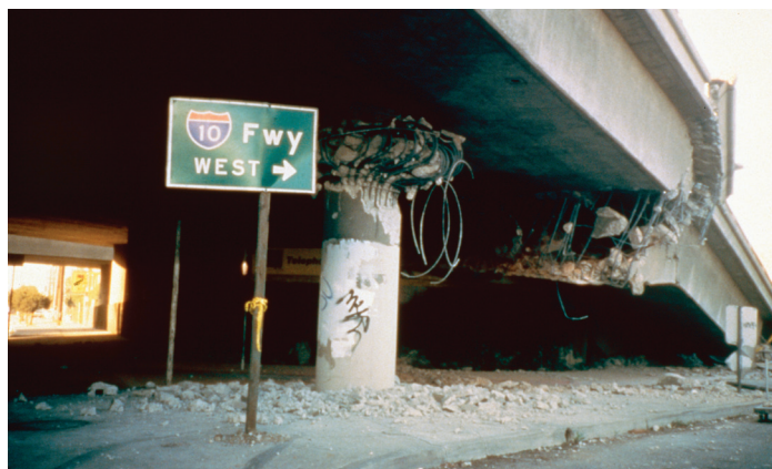
Collapse of the Interstate-10 overcrossing structure at Venice and La Cienega boulevards.
