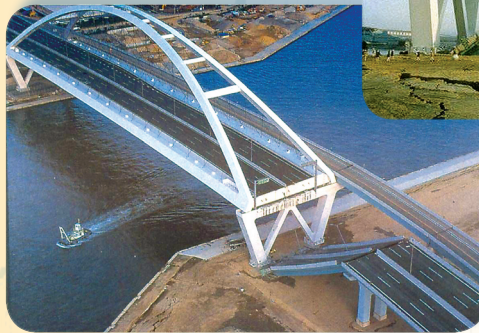
Two views of a collapsed segment of the Nishinomiya Bridge due to soil liquefaction and lateral spreading after the 1995 earthquake that struck Kobe, Japan.
