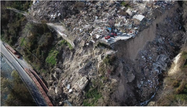
Aerial photograph of the 2016 landslide that impacted Strada Statale No 4 below Pescara del Tronto
